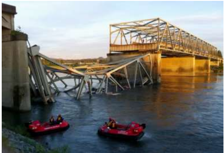
Figure 3-8 Skagit County Bridge Collapse
