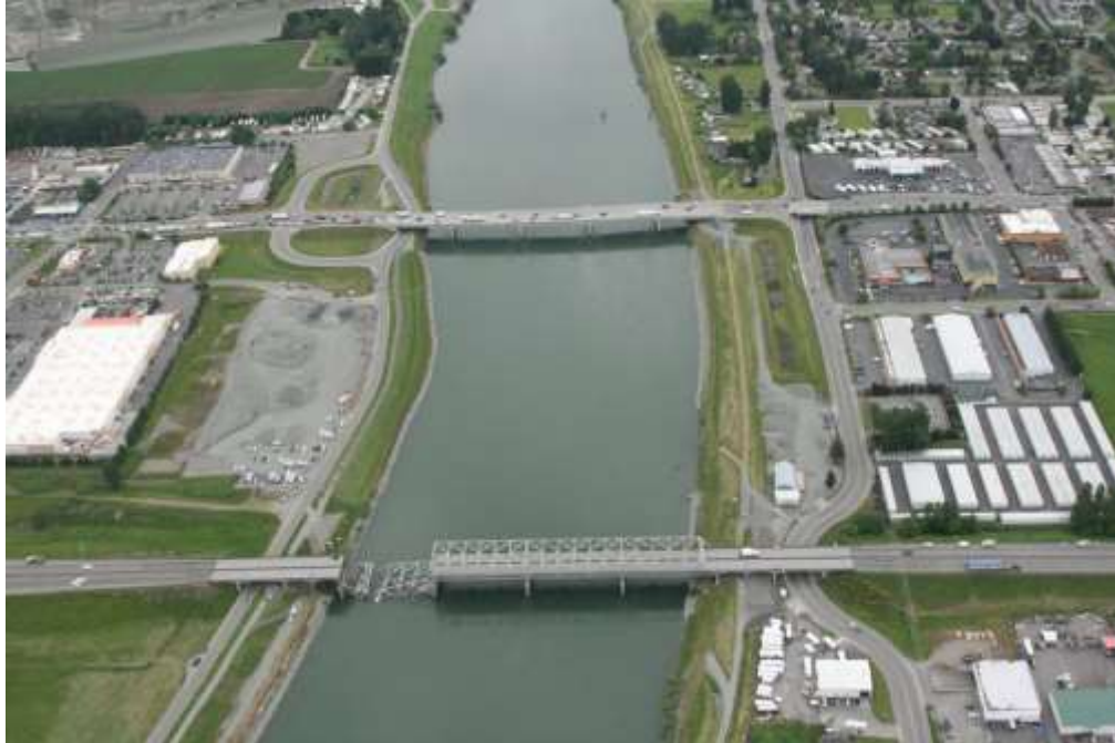
Figure 3-9 Extended View of Skagit County Bridge Collapse
